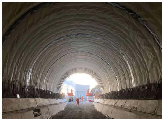
Mined Tunnel (drained) + Cross-passage, Switzerland, SikaProof®-200, 30,000 m 2
