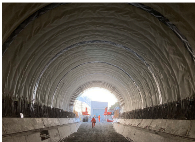
Mined Tunnel (drained) + Cross-passage, Switzerland, SikaProof®-200, 30,000 m 2
