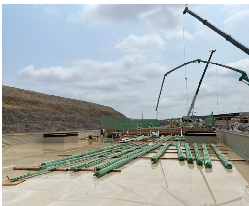
Cut & Cover Tunnel, Airport Tunnel, USA, Pre- & Post-applied SikaProof® A+, 10,000 m 2
