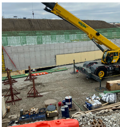
Cut & Cover Tunnel, Airport Tunnel, USA, Pre- & Post-applied SikaProof® A+, 10,000 m 2
