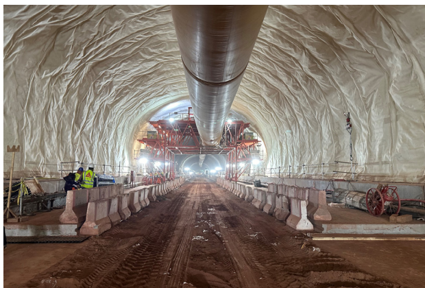
Mined Tunnel (drained), Saudi Arabia, SikaProof®-110, 1,000,000 m 2
