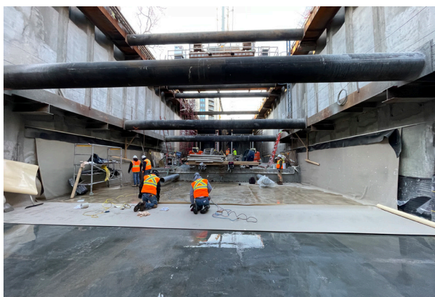
Cut & Cover Tunnel, LRT Tunnel, USA, Pre- & Post-applied SikaProof® A+
