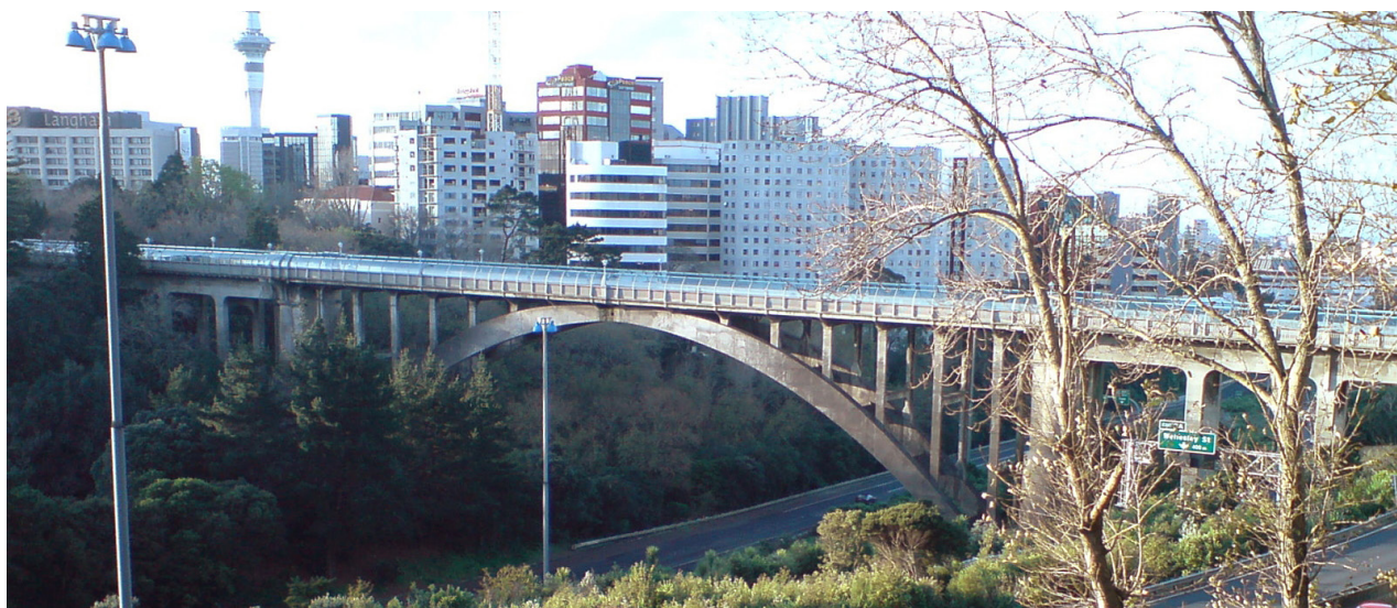
Grafton Bridge, Auckland, New Zealand
