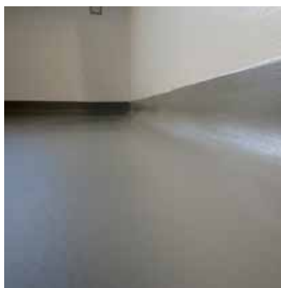
Sikafloor® FLOOR-WALL COATING CONNECTION WITH RIGID COVE
