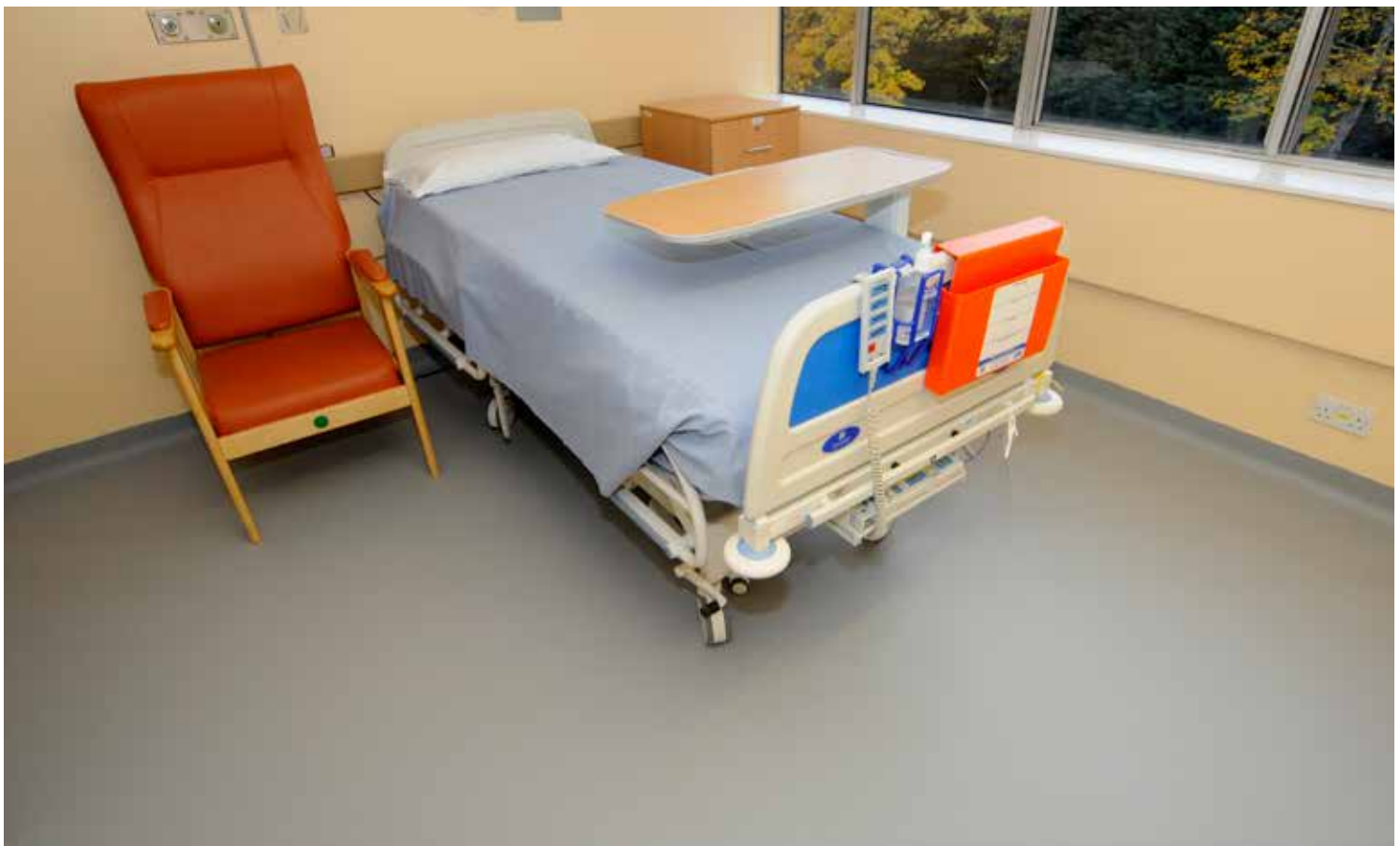
Sika's standard Sika® ComfortFloor® flooring installed in a refurbished single room at York Hospital, UK.
